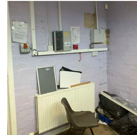
EXISTING INTERNAL PHOTOS
