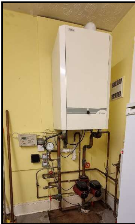
Figure 2 – Gas Boiler
