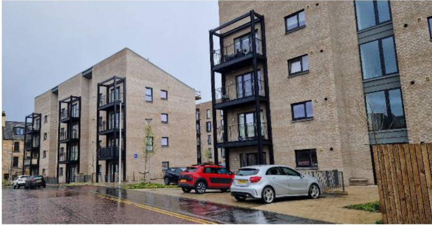
Link/C-urb Housing Association, social rented General and Particular Needs, Paisley Town Centre
