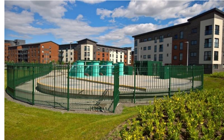
Construction of Phase 3 - North Renfrew Flood Prevention Scheme Pumping Station
