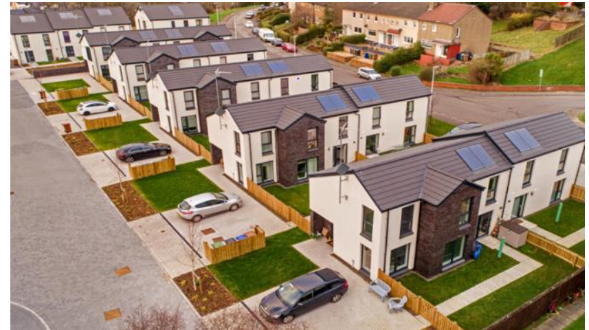
New build social rented housing, St Ninian's Crescent, Paisley (Link Group)
