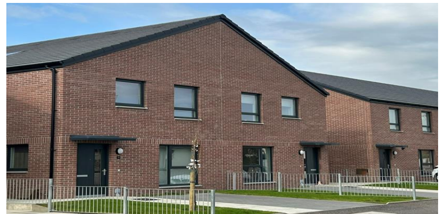
New build social rented housing, Albert Road, Renfrew (Williamsburgh Housing Association)
