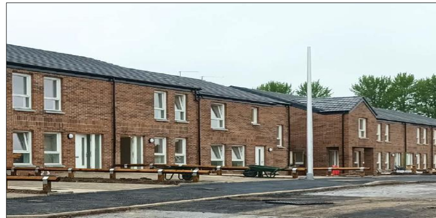
New build Council Housing for social rent, Auchengreoch Road, Johnstone
