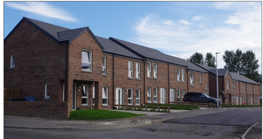
New build Council Housing for social rent, Auchengreoch Road, Johnstone
