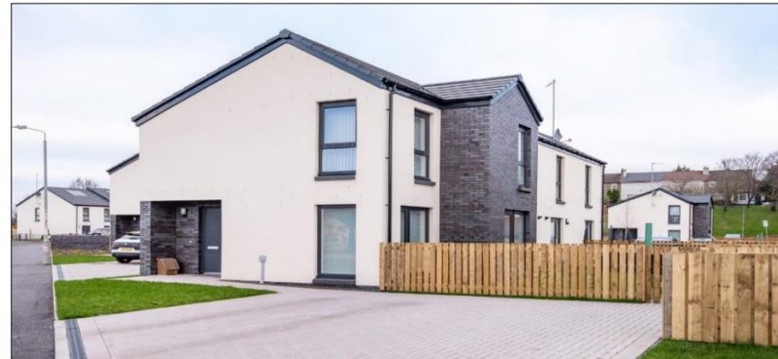
New build social rented housing, St Ninian's Crescent, Paisley (Link Group)
