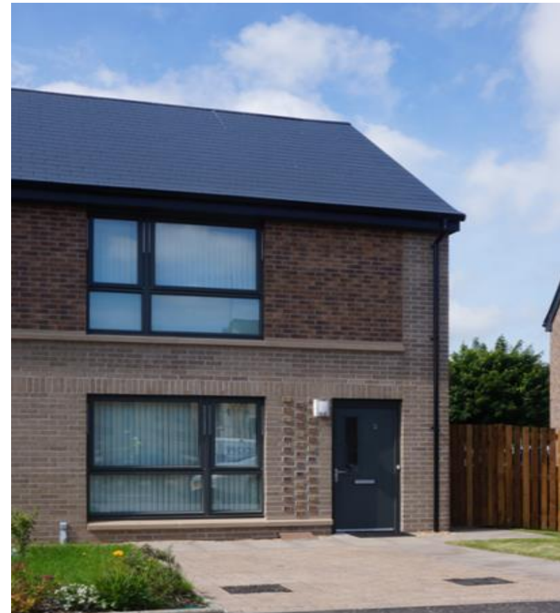
New Affordable Housing development in Renfrew, Sanctuary Scotland
