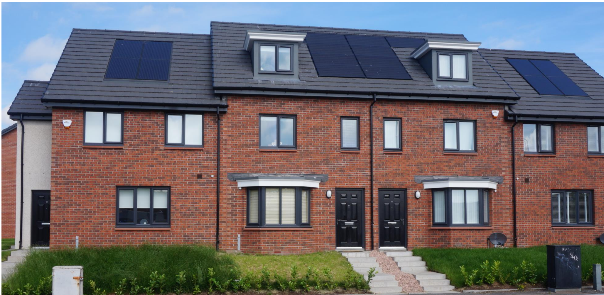
Renewable technology used in new housing development at Shortroods, Paisley
