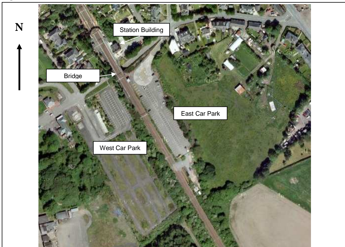
Figure 1.1 Current Park and Ride facilities
