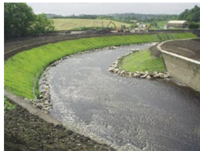
Crosslee Flood Prevention Scheme
