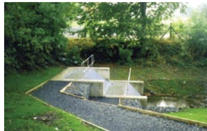
Amochrie Road Culvert and Inlet Screen
