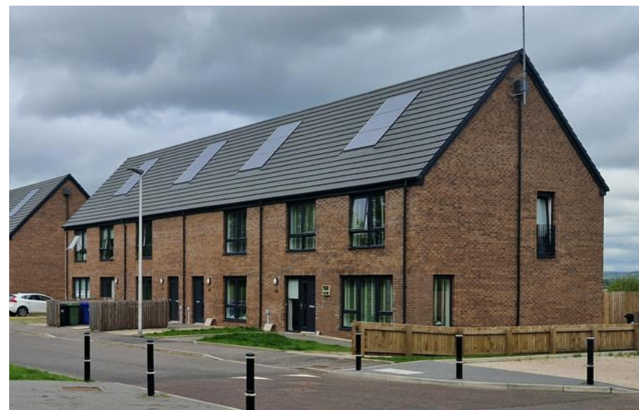
New build social rented housing, Millarston, Paisley, (Link Group)
